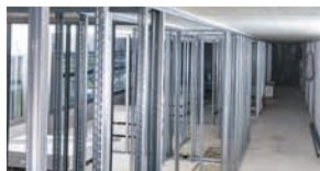
Drywall tracks to concrete and steel
